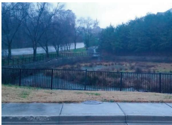
**Figure 1: Wet pond with permanent pool storage and temporary detention in a residential setting (Source: SMART Center).**
