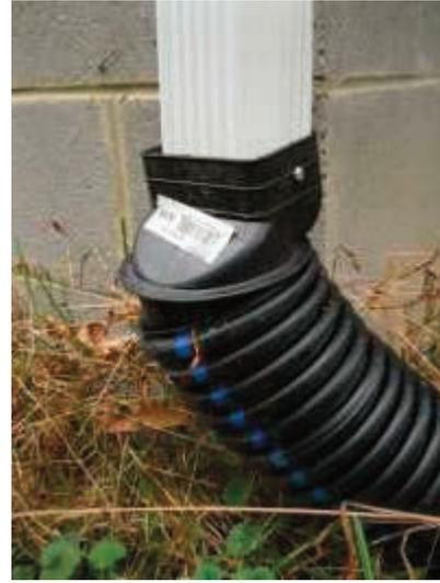
**Figure 3: Disconnected downspouts on the left and a converter joint on the right (Source: Carmen, NCSU).**
