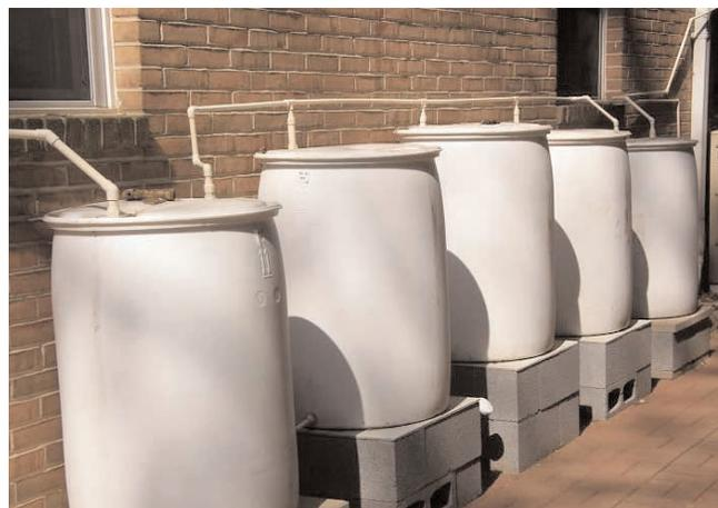
**Figure 2: Set of rain barrels (Source: VADCR, 2011).**
